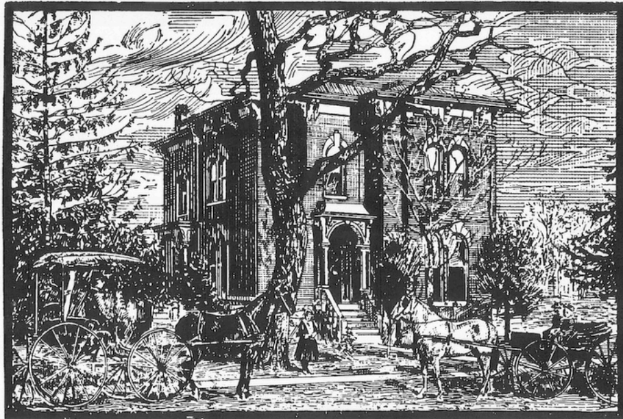
M. CALMER'S RESIDENCE.
